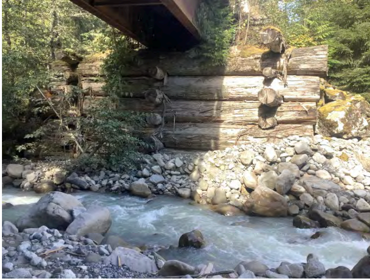
Right Bank Abutment when facing downstream
