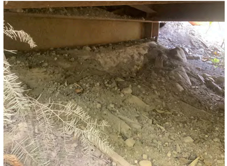
Right Bank Abutment when facing downstream
