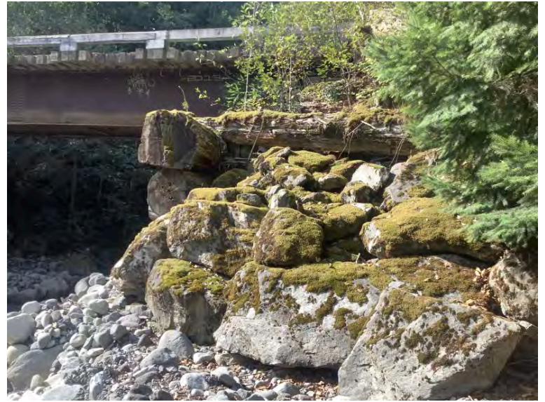
Right Bank Abutment when facing downstream
